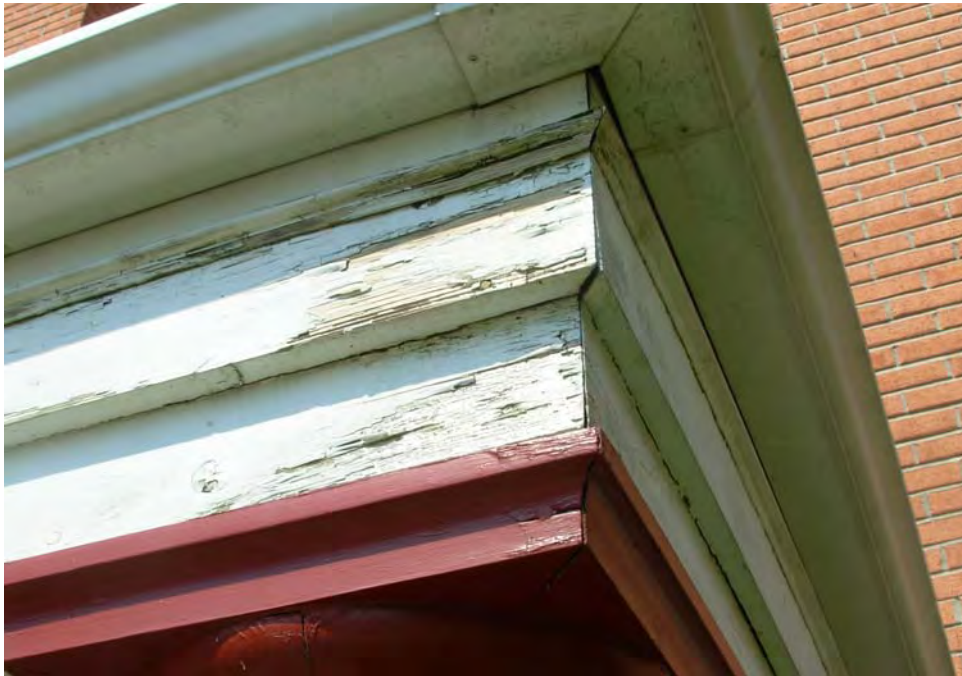
3. Wood trim deterioration at entrance canopies
