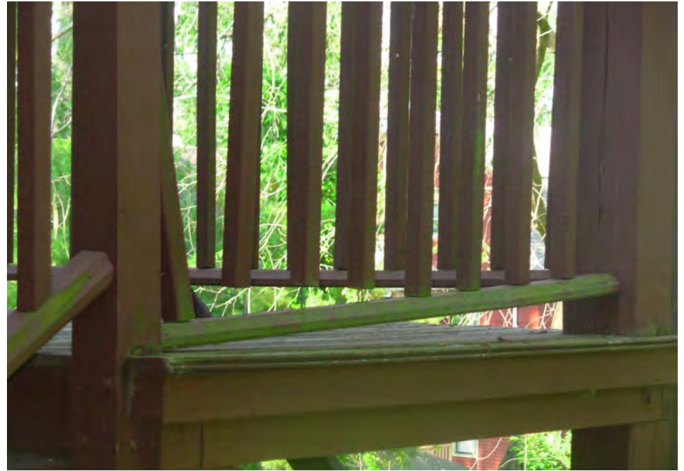
6. Railing damage and deterioration at balconies
