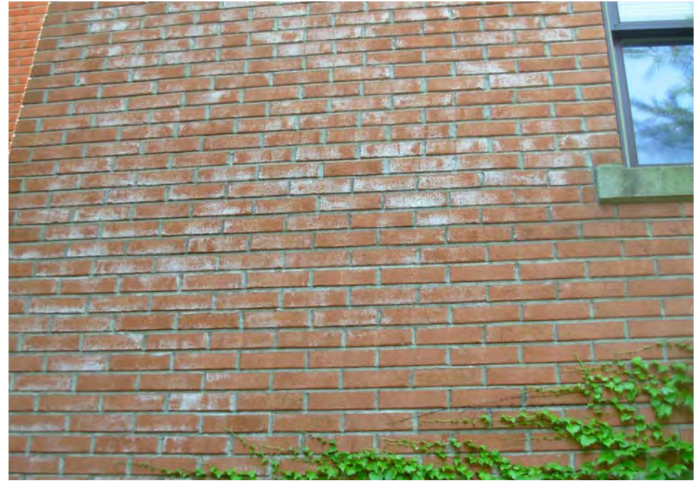
2. Brick masonry efflorescence, minimal mortar deterioration
