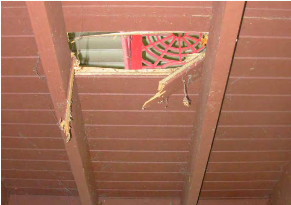
7. Hole in decking at rear balcony of 49 Vine Street
